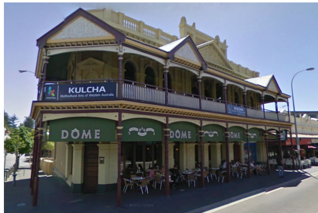
1899 Literary Institute (fmr), 13 South Terrace, Fremantle by Wilkinson Smith & Wilson (Google 2012)
